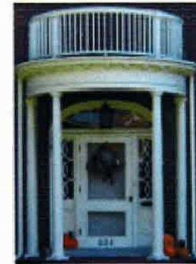
SHALLOW PROJECTING CENTRAL FACADE
