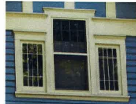
VERTICAL MUNTINS / INTERMEDIATE JAMB BETWEEN WINDOWS
