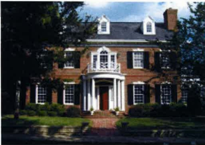
HISTORICAL GEORGIAN ARCHITECTURE
