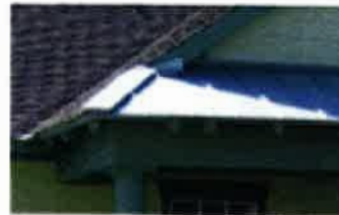
METAL ROOFS / EXPOSED RAFTER TAIL
