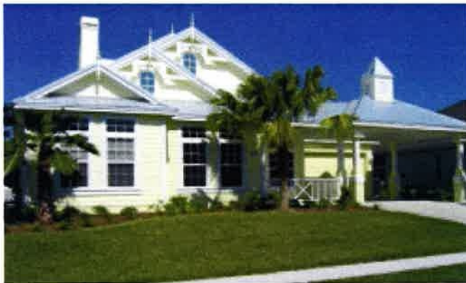
BATTERED COLUMNS / MULTIPLE ROOF PLANES
