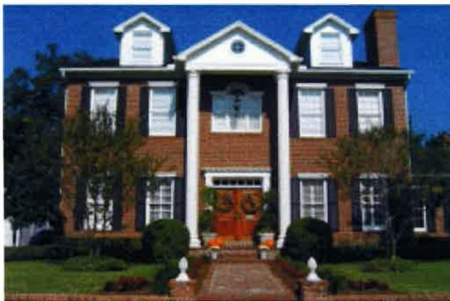
2 STORY BRICK / DENTILS AT CORNICE
